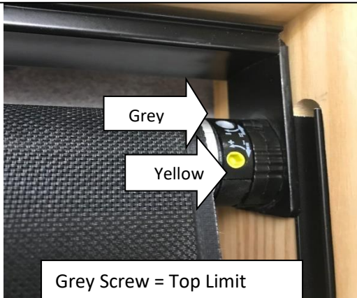
Image 3: Motor on the right side and fabric drops towards the front of the roller
