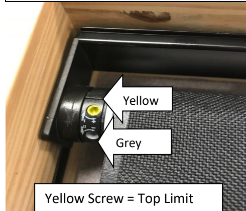
Image 2: Motor on the left side and fabric drops towards the front of the roller
